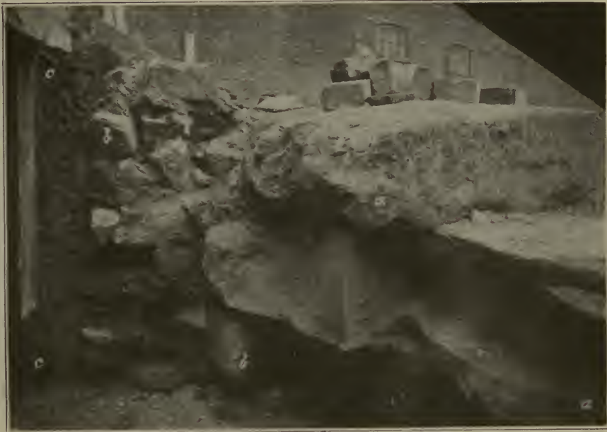
FIG. 5.—ROMAN WALL (INTERIOR, LOOKING NORTH). a Inner face of Ashlar work ; b Rubble ; c Clay-loam backing.
